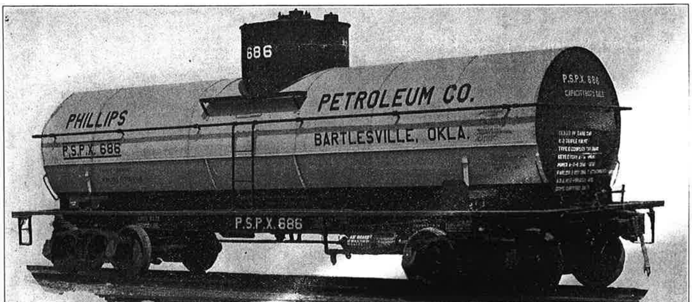
A. R. A. Class IV Tank Car Built by the General American Tank Car Corporation for the Phillips Petroleum Co., Bartlesville, Okla.
